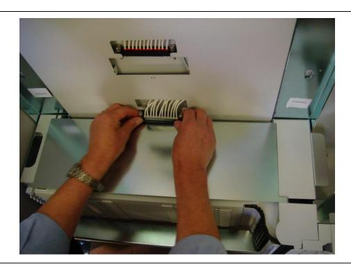
• Insert Male Connector block from rear panel of OCR Rack into the Female Connector on the Sub Rack. Fully tighten the 2 thumb screws to lock the connectors together. Installation of the sub rack is now complete.
