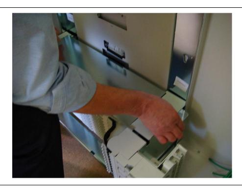
. Move Sub Rack Assembly into position in OCR Rack.
