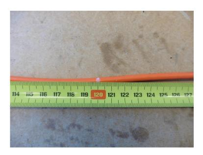
• Make a marker where the Closure should be installed. Make sure it is at least 1.2 meter to the end of the cable.
