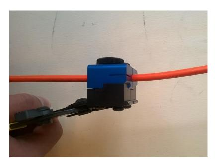
• Use Ripley stripping slitter to open the cable out sheath along the length direction, from the marker to the end of the cable.
