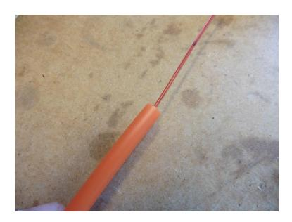
• Make sure the end surface of micro duct is flat.
