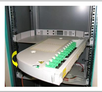
• Swing out the Splice and patch Module to fully open.
