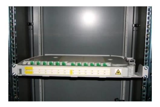
• Using four, M6 x 12mm screws (8) fit shelf in position.
