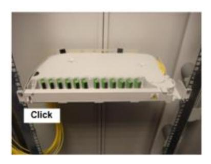
Push the shelf back into the closed position. Push this fully back into the shelf a click will be heard when the locking tab has been engaged on the metalwork.
