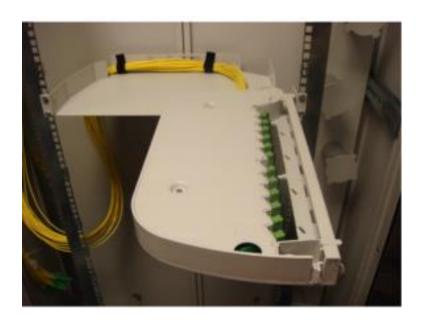
Replace the cover making sure that it sits flat and is recessed correctly. Replace the 2 M4 screws which were removed in Step 5.
