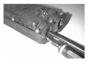
De-pressurize the box by depressing the valve in the top cover.
