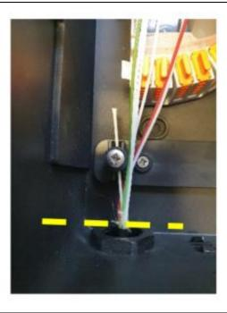
• Strip 1.2m of input cable as required and feed through gland, ensuring the cable butt is as close to the end of the gland as possible.
