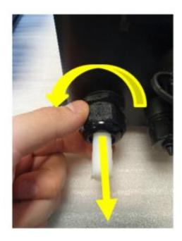
• Remove blank from input cable gland as required.
