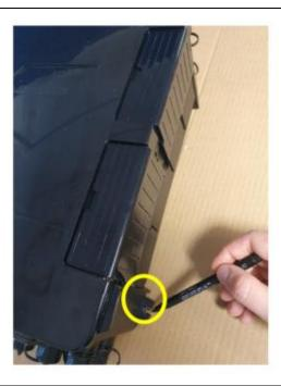
• Ensuring the box is straight, mark and drill the final 2 positions on the side of the box and fit the final 2 screws.
