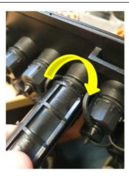
• Tighten the shroud nut fully using the port tool provided.
