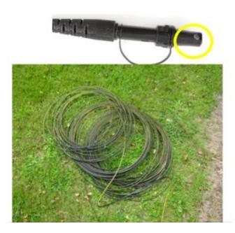
• Pull the cable from the customer end through the duct to the closure using the pulling eye on the connector.
